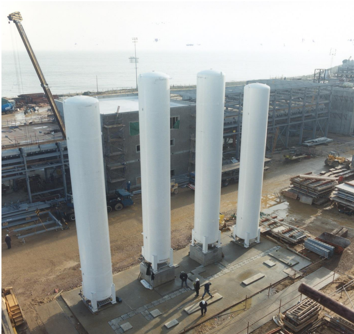
Low Pressure Nitrogen Storage Tanks
